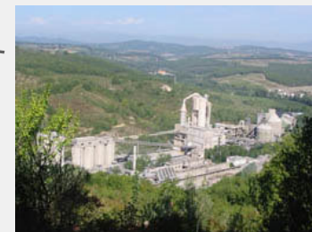
Greve in Chianti (FI) Full-cycle cement plant
